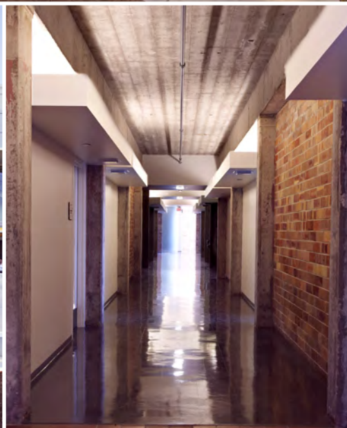
Architectural concrete walls, floors, stairs and roof overhangs complement the concrete of the original building and bring new character to the building circulation spaces.
