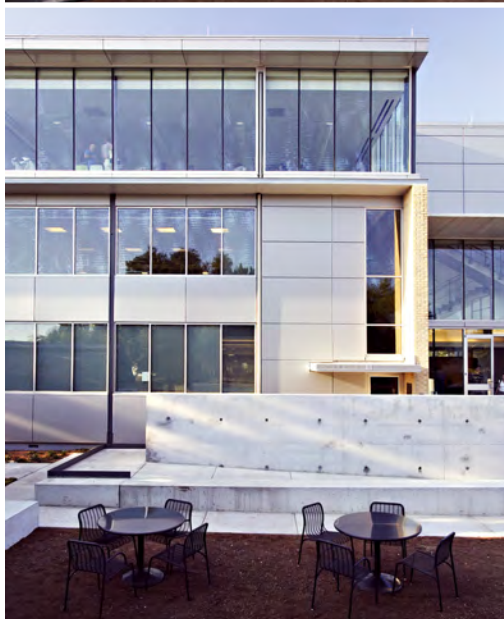
Architectural concrete walls, floors, stairs and roof overhangs complement the concrete of the original building and bring new character to the building circulation spaces.
