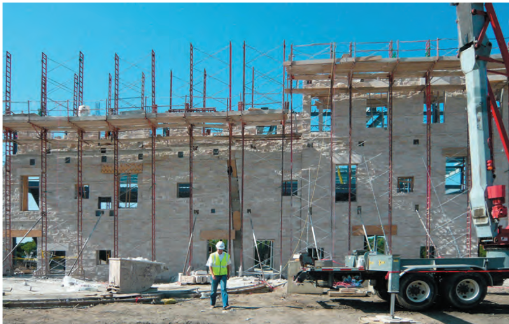
An innovative system of load-bearing masonry wall construction singularly incorporates structural support, thermal insulation, and moisture protection within a unique double-wythe masonry cavity wall.
