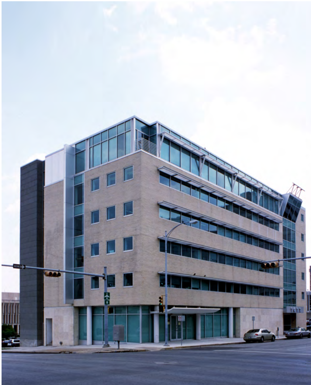
The single wythe AAC wall, only eight inches thick, provides a four hour fire rating, effective thermal insulation and a durable, attractive exterior finish.
