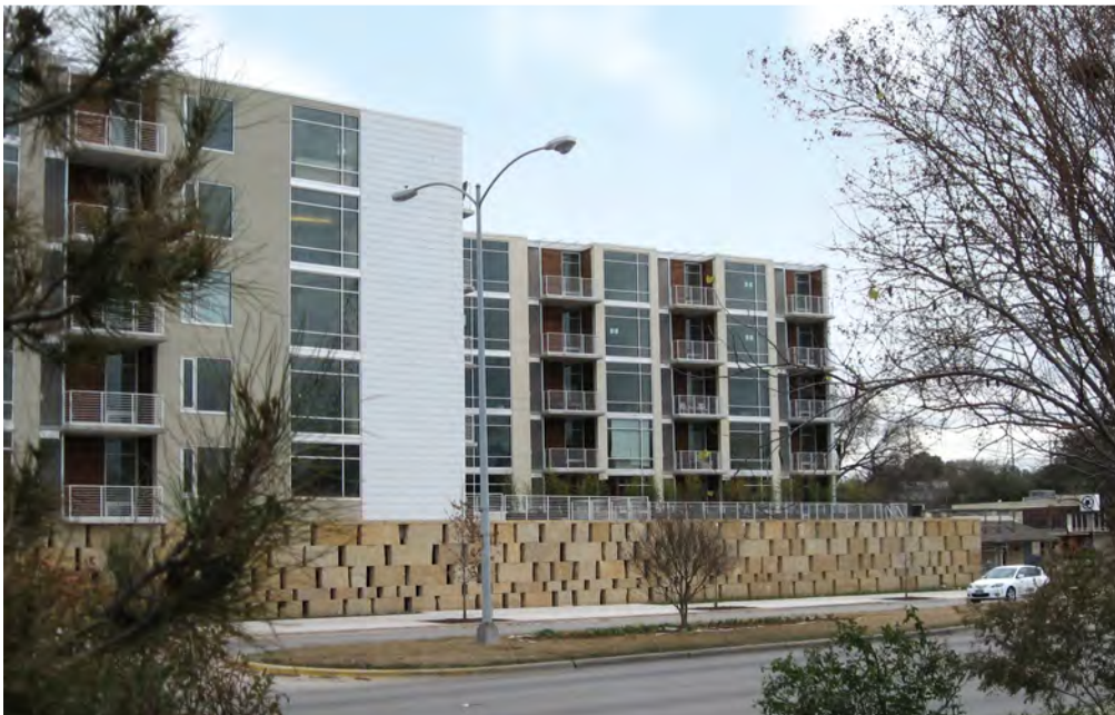
A perforated, stacked limestone wall buffers the building from busy Lamar Street traffic.
