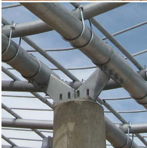
Galvanized steel pipe and round bars form the vocabulary of the Lake Park structures.
