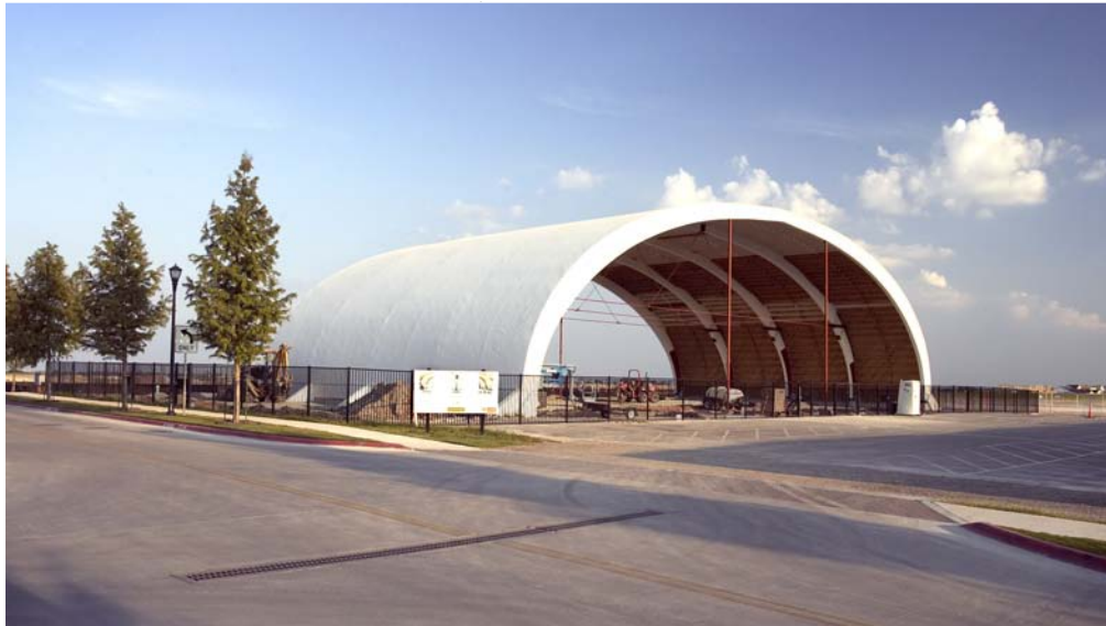
White paint demarcates original lumber in the arches and roof deck. Clear-coated pine delineates new replacement lumber. Red paint identifies new steel reinforcement of the arch bases and the addition of an arch tie, originally added in the 1970's and revised in the present renovation.
